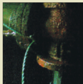
A reservoir ballcock held in place by a rope is just one of numerous items requiring replacement on our GWS.
