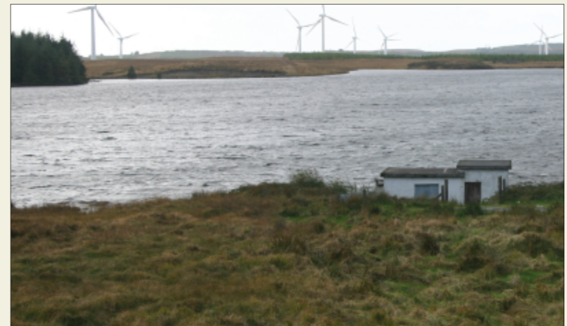
Deteriorating raw water quality in Loch na Minna in 2008 had an impact on treated water quality. A proposal is now on the table to enhance the treatment plant facilities so that a quality treated supply can be guaranteed, even with difficult raw water.
